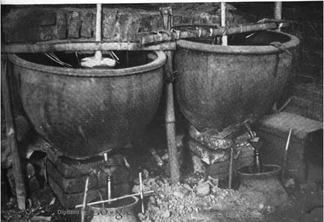
(Top) Production of cananga oil in the Bantam region of Java (Indonesia). Primitive direct fire stills serve for the distillation of the flowers. (Bottom) Cananga oil, Bantam region. View of primitive condensers and oil separators. Photos Fritzsche Brothers, Inc., New York.
