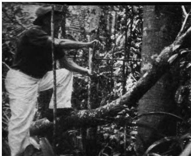
(Top) Production of balsam copaiba in the lower Amazon Basin, State of Pará, Brazil. A hole is drilled into the lower part of the trunk, from which the balsam will flow. (Right) Production of balsam Peru in El Salvador, C. A. "Cascara Process": Incisions are made in the trunk of a tree, after it has been scorched with a torch flame. (Bottom Left) Balsam Peru, El Salvador, C. A. "Trapo Process": Burlap is hammered into the incisions to absorb the flowing balsam. (Bottom Right) Balsam Peru, El Salvador, C. A. "Trapo Process": A bundle of burlap soaked with balsam and removed from the incisions. Photos Fritzsche Brothers, Inc., New York.
